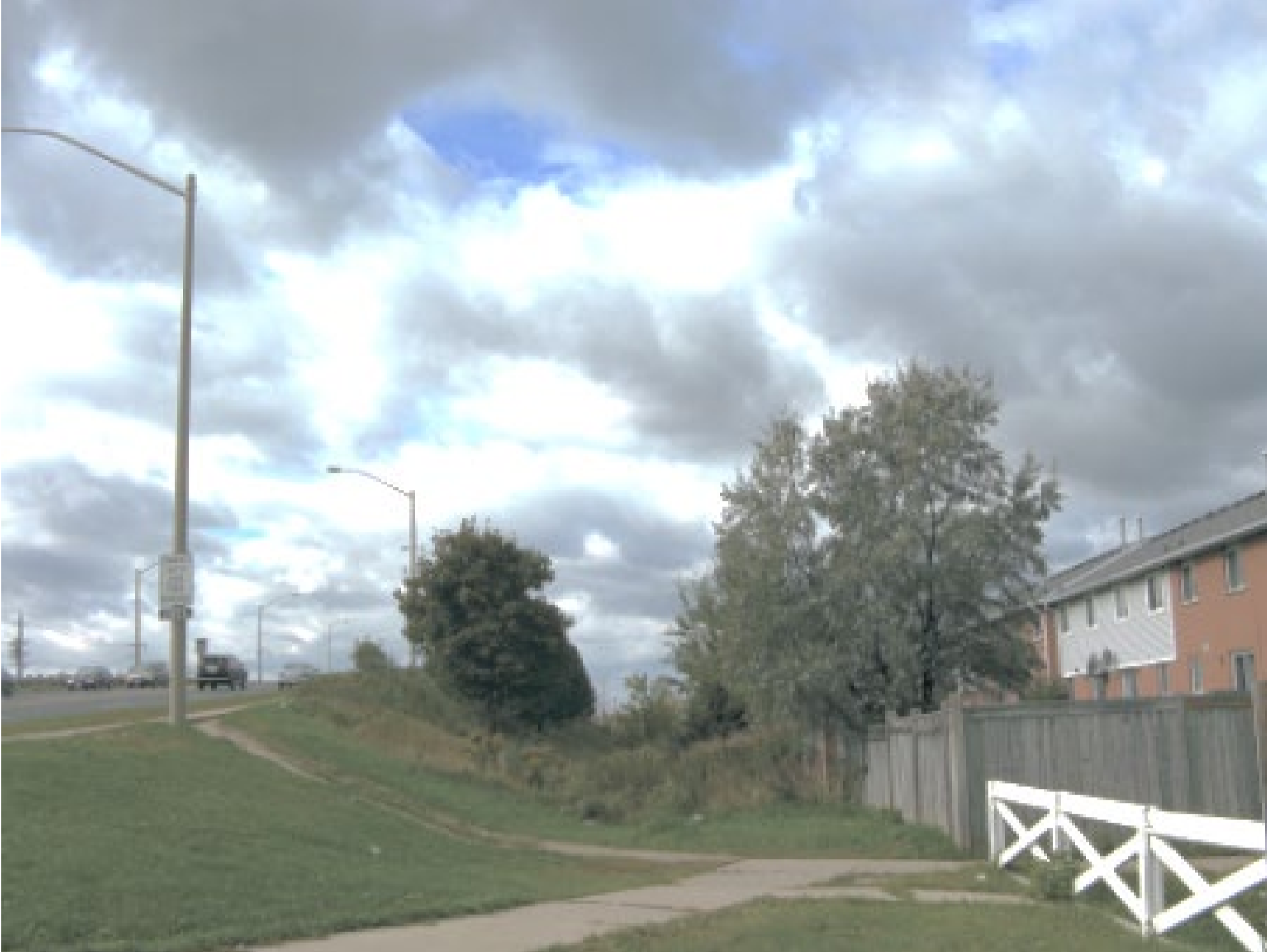
Bayview Avenue south of Highway 407
