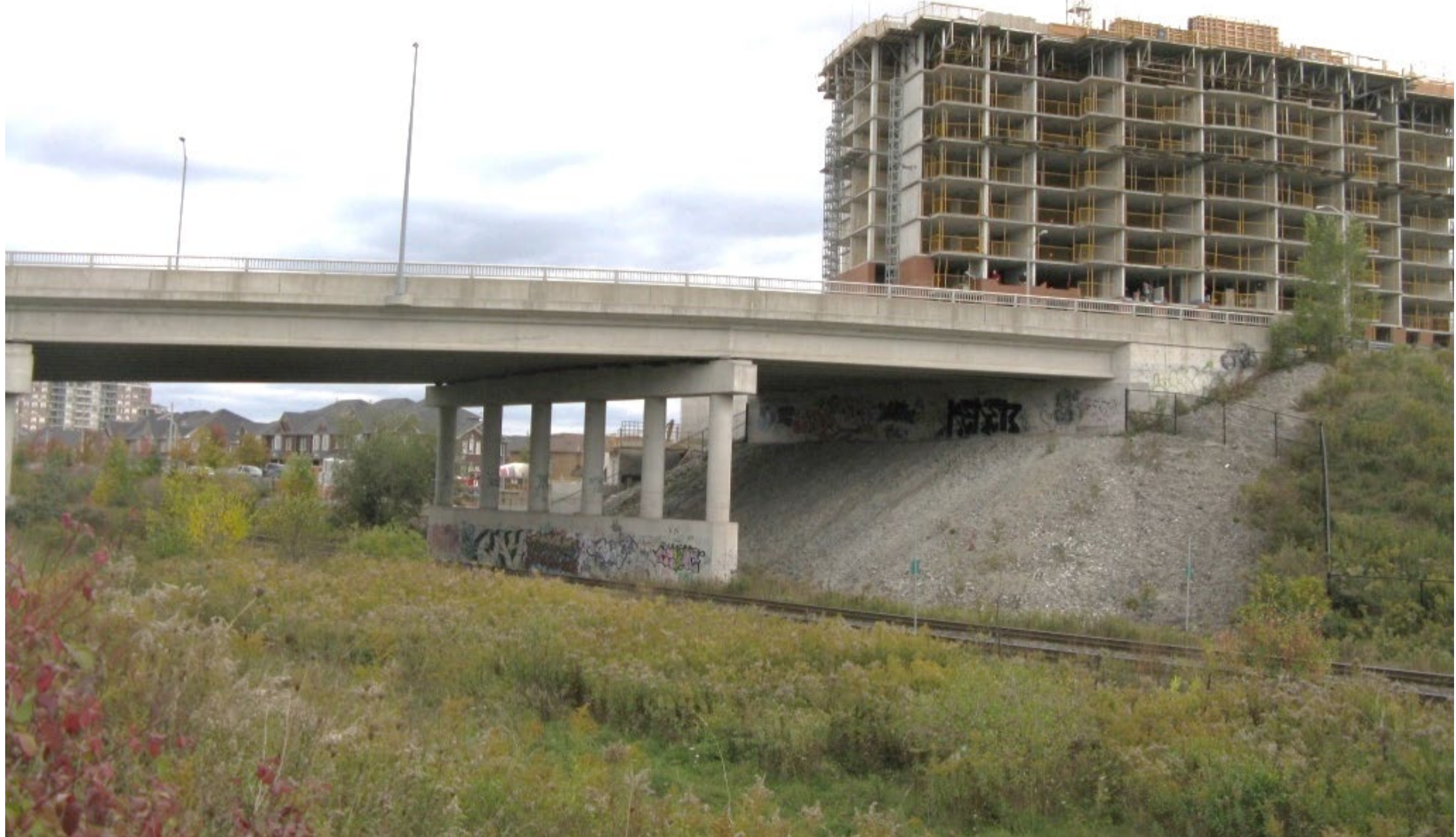
Bantry Avenue east of Yonge Street
