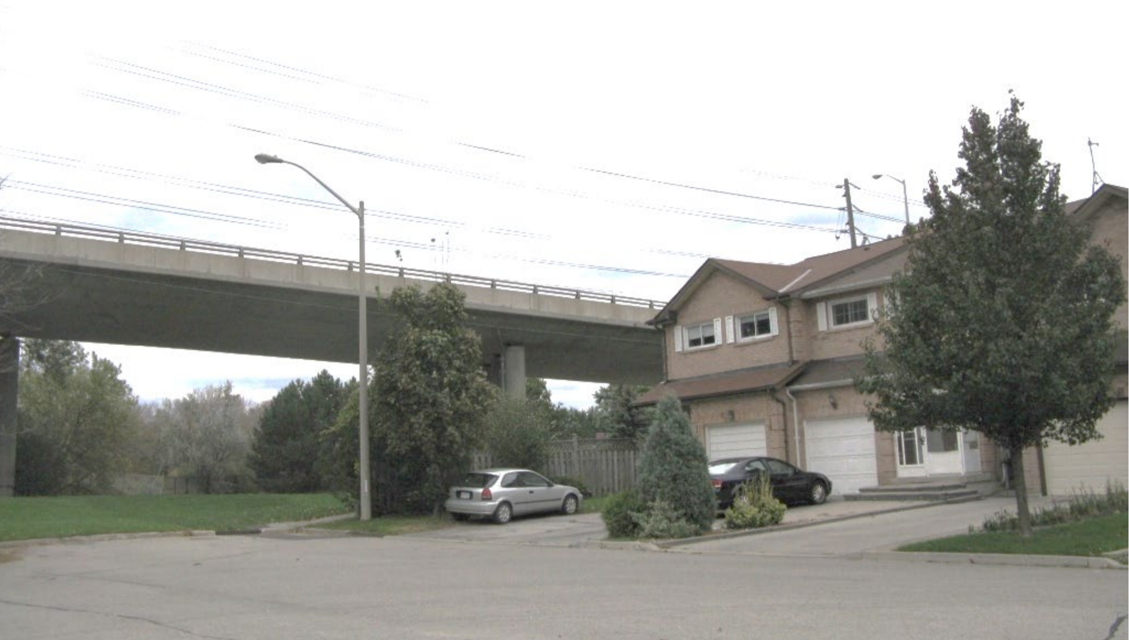
Bayview Avenue south of Highway 407
