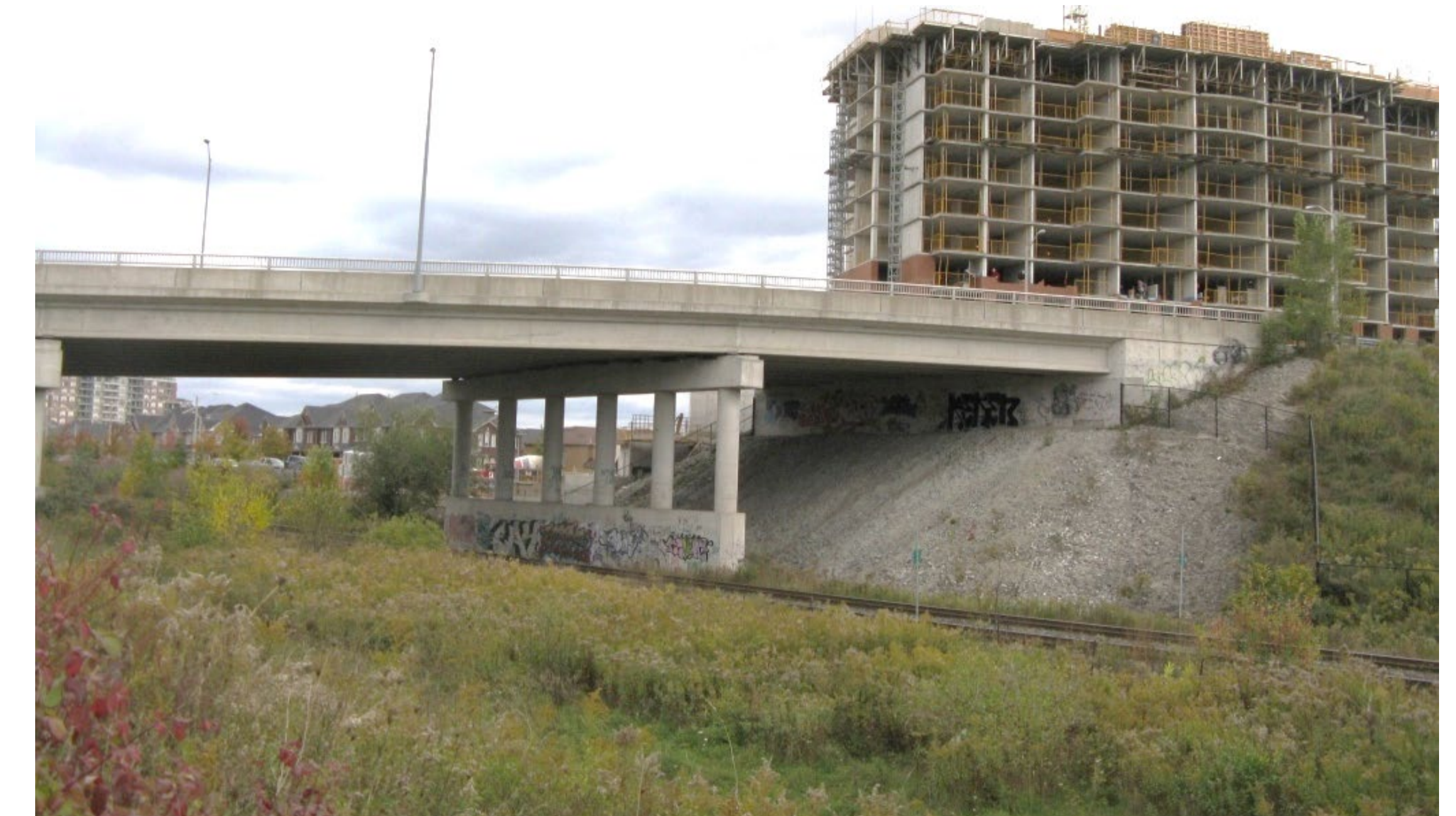
Overpass Example: Bantry Avenue east of Yonge Street
