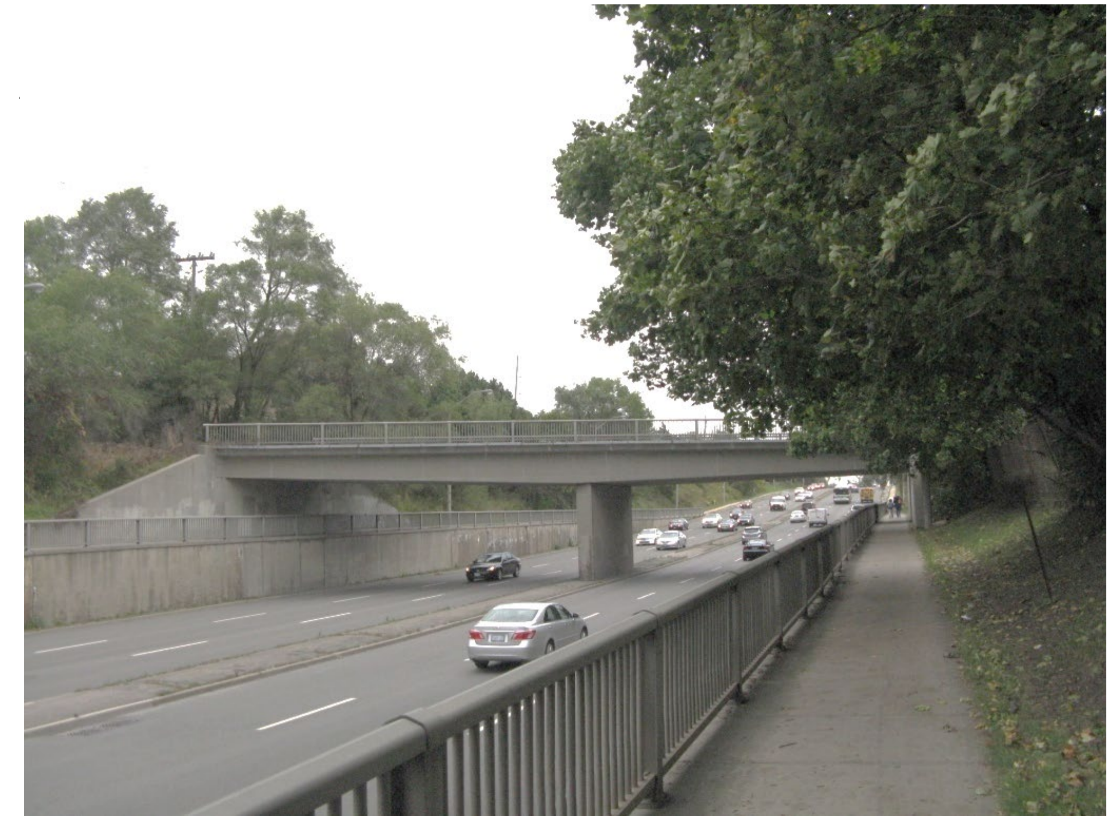
Underpass Example: Steeles Avenue west of Leslie Street
