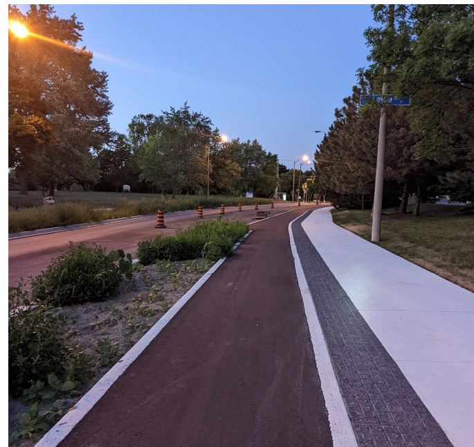
Bundled state of good repair and cycling project on Cummer Ave., including a green buffer separating the cycle track and sidewalk from vehicular lanes.
