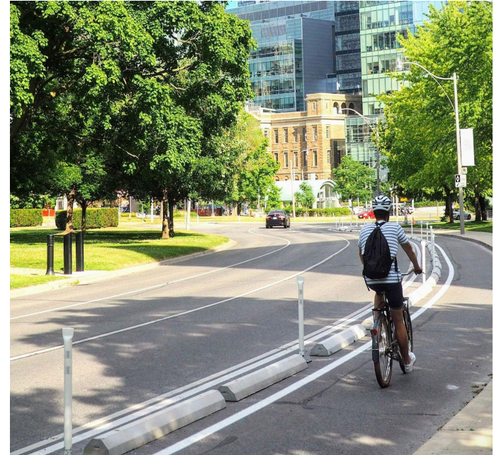
An example of materials that can be used in quick-build projects, including pavement markings, precast concrete curbs and bollards.
