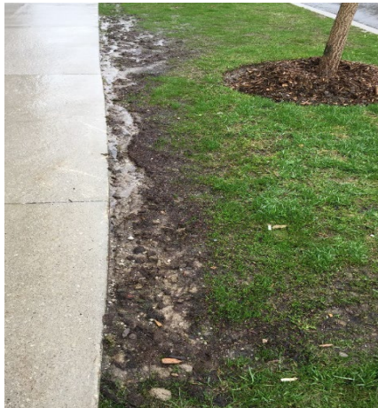
Example of eroded barrier
