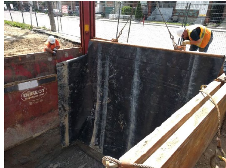
Liner installation to prevent migration
