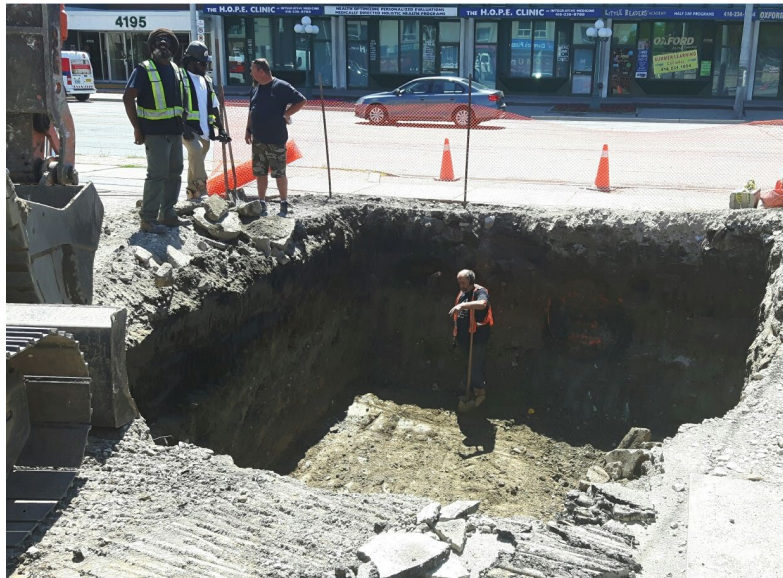
Example of Excavation and UST
