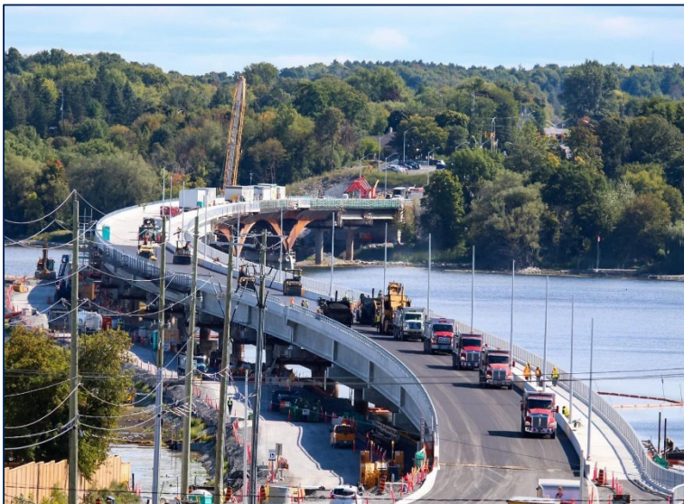
Third Crossing, City of Kingston
