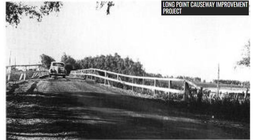
The Causeway was constructed with wooden bridges. The longest bridge spanning Big Creek is shown here.
