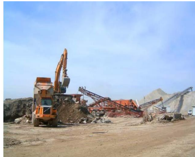
Pearson International Airport – On Site Concrete Crushing Plant and Processed Concrete Backfill (2004)
