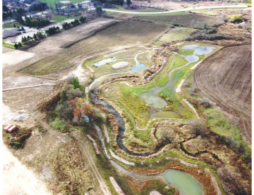
Stoney Creek Flood Control Facility, London, ON
