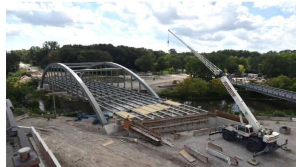
CITY OF LONDON - The Victoria bridge replacement project in London, Ont. not only replaces an older structure but also ensures the crossing can better withstand the effects of climate change. The new through-arch steel structure removes the need for a central pier mid-river that often snagged debris at times of high flows.
