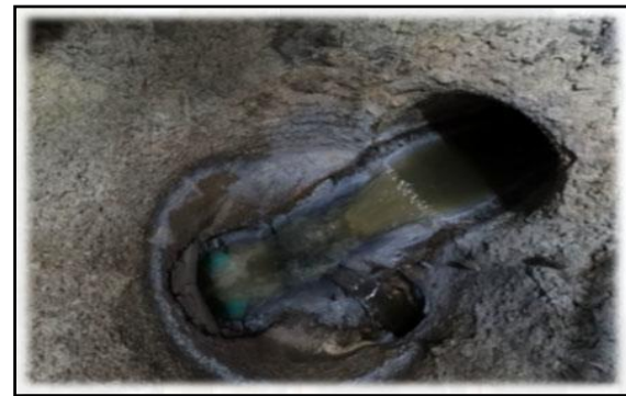
Picture 2: Hydrogen Sulfide Damage
