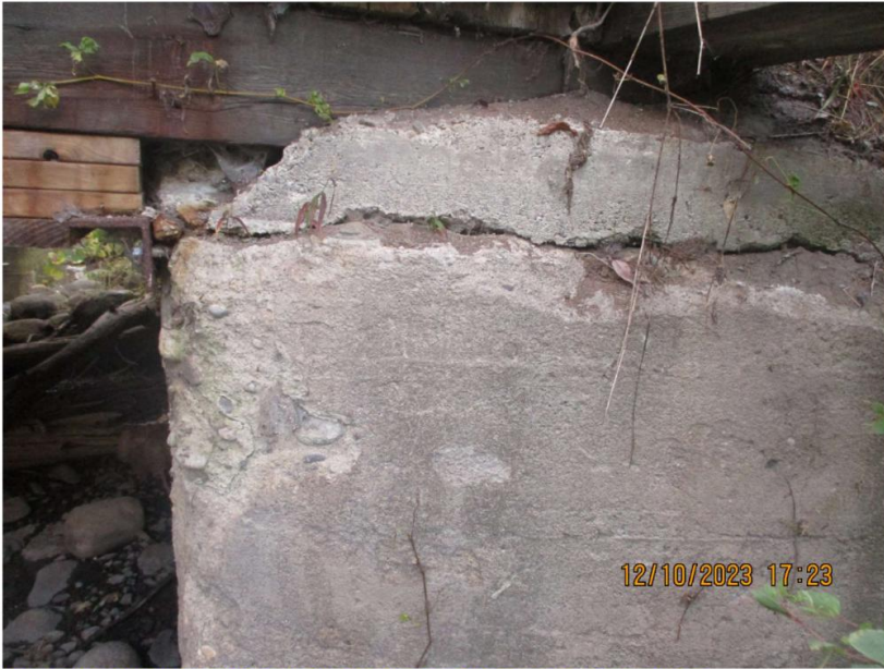
Figure 30 : Northeast Wingwall_Evidence of Severe Disintegration.
