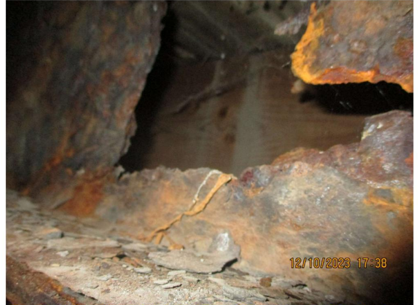
Figure 34 : Stringer I beam North End_Evidence of Severe Corrosion & Section Loss.
