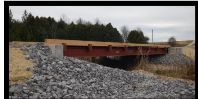
Photo 6: Upstream face of new 15.2m span x 6.1m wide Lessard Modular bridge.
