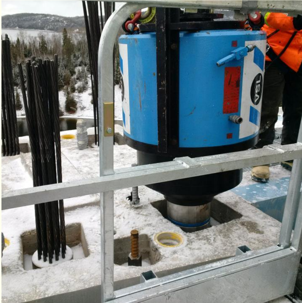
Towers have both temporary and permanent PT
