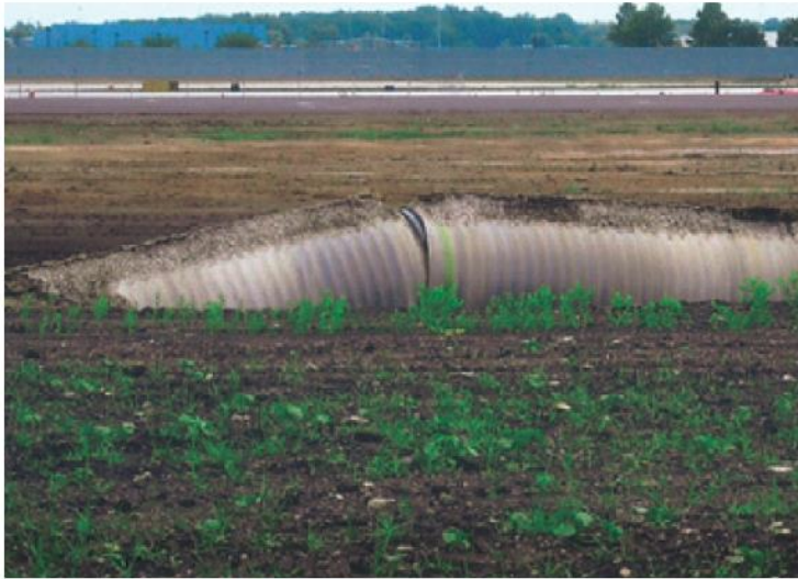
Columbus, Ohio Airport – polypropylene pipe floating out of ground
